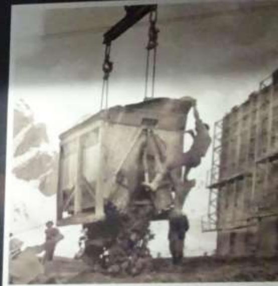
A worker opening a container with subcrete.
